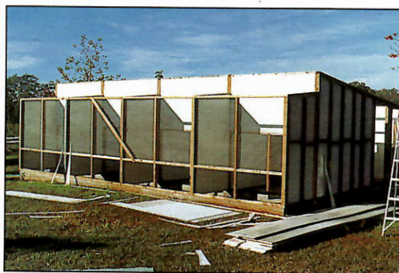
Right: Front view showing the shield walls to protect enclosed areas.
