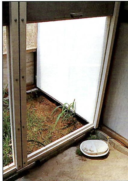
Right: Internal sliding shutters to provide winter protection. Below: Front view of the finished aviary.
