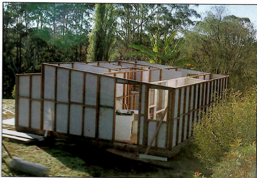
Below: Internal walls and partitions lined with Hardiflex.
